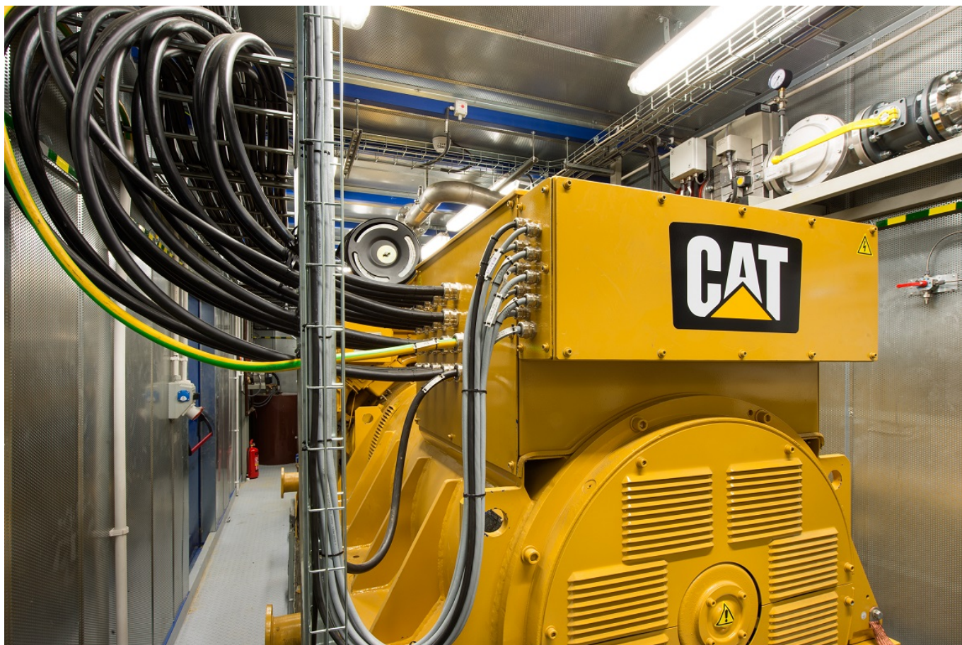
Model agregatu: CATERPILLAR CG170-12 Moc: 0,99MWe
